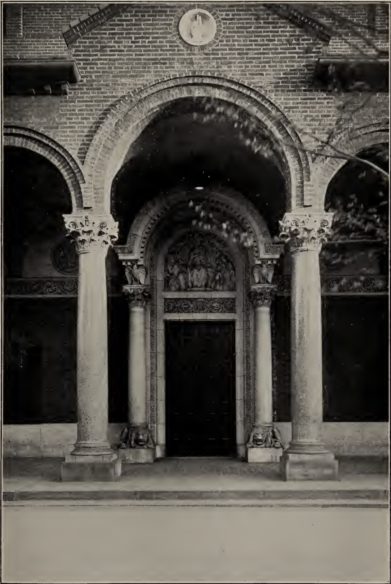
MAIN ENTRANCE The Church of the Nativity of Our Blessed Lord
